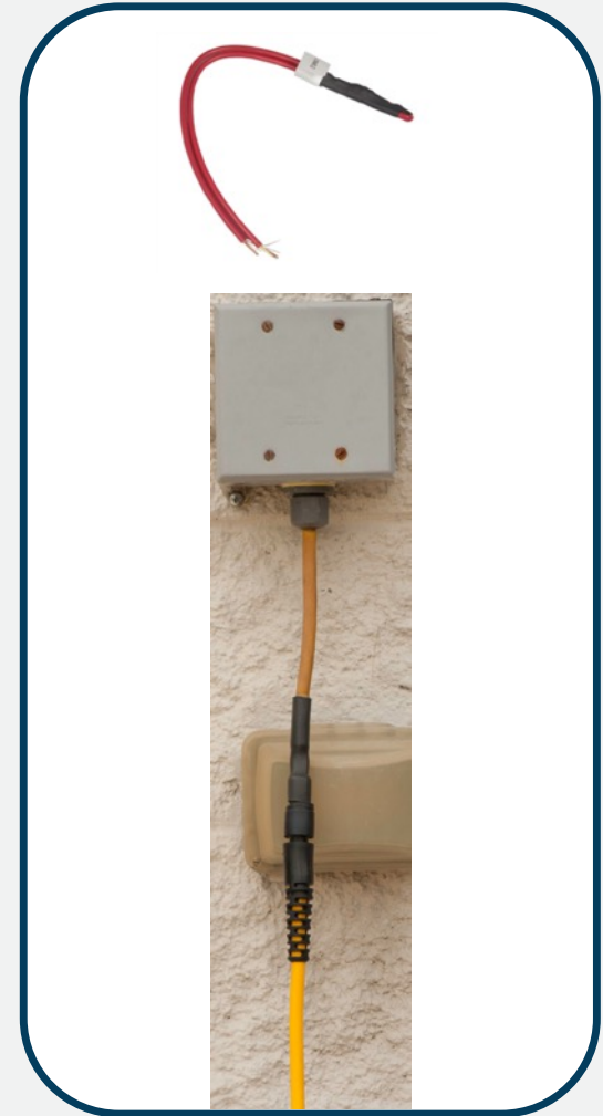
FINISH BY SPLICING AN EOL RESISTOR
